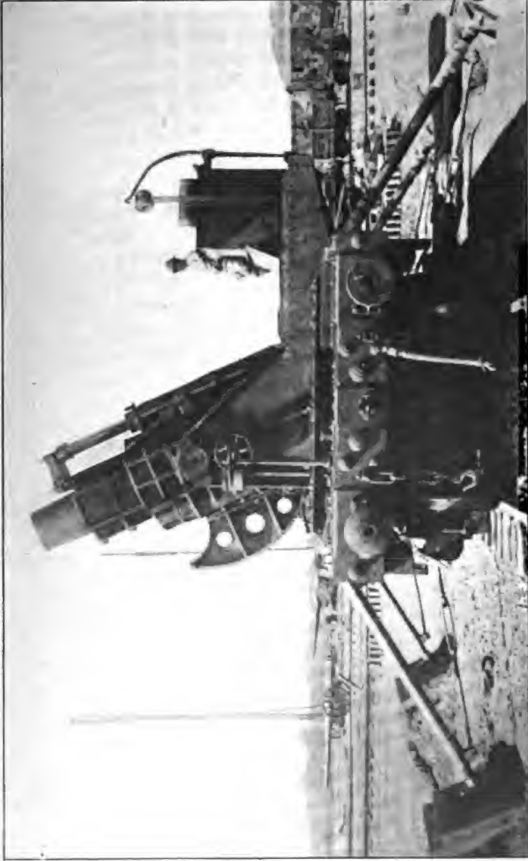
12-INCH AMERICAN MORTAR ON RAILWAY MOUNT.
